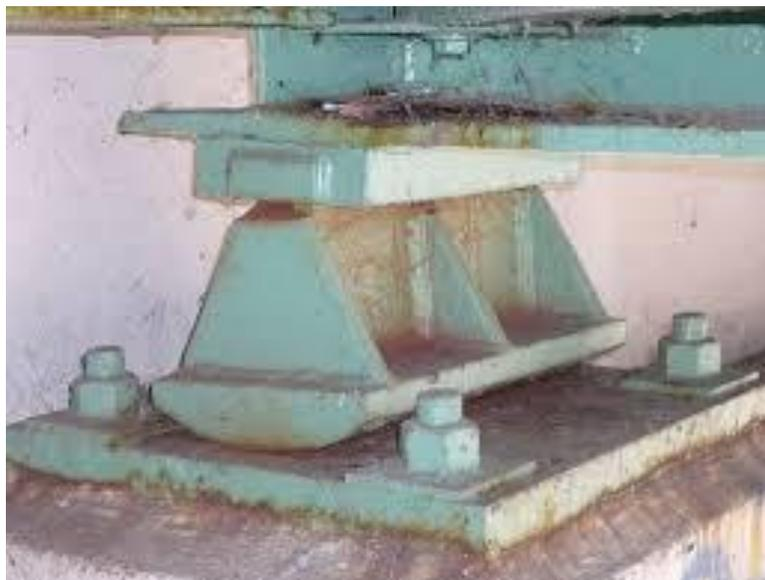
*Fig 7 Rocker Bearing*
